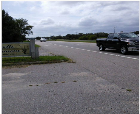
Looking south from Eastville Commons
