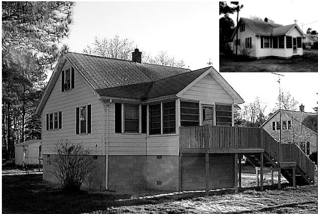
PICTURE 8.2 The county elevated this home using Hazard Mitigation Grant Program money. Photos by David Fluhart
